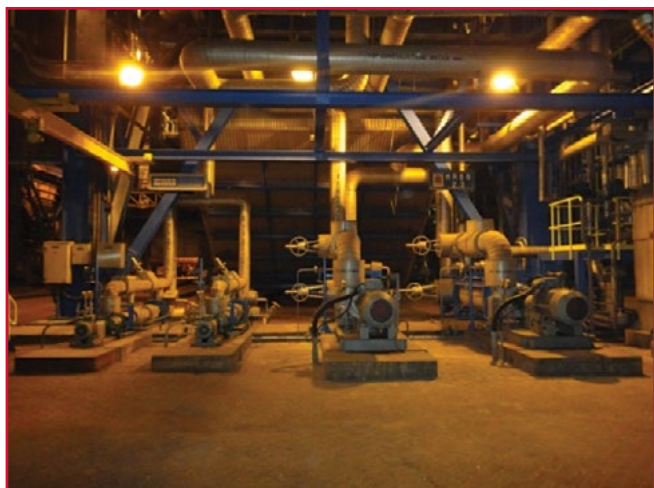
High Pressure Sodium Lighting
